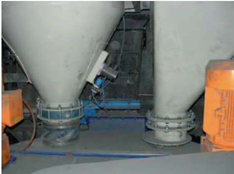
Loosening hard crusts with pneumatic linear vibrators
