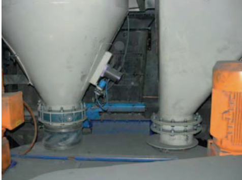
Loosening hard crusts with pneumatic linear vibrators
