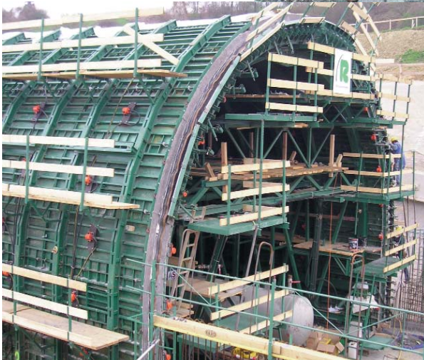
Tunnel formwork with pneumatic external vibrators from the NVT series
