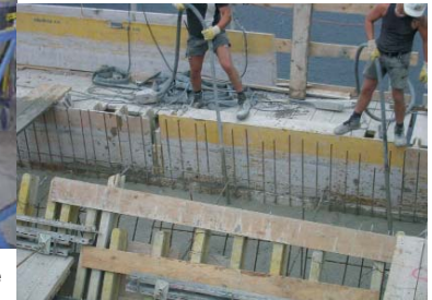
Compacting concrete in a building, using electric internal vibrators from the NCZ series
