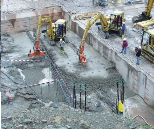
Excavator equipped with hydraulic internal vibrators from the NHR series, for compacting bulk concrete
